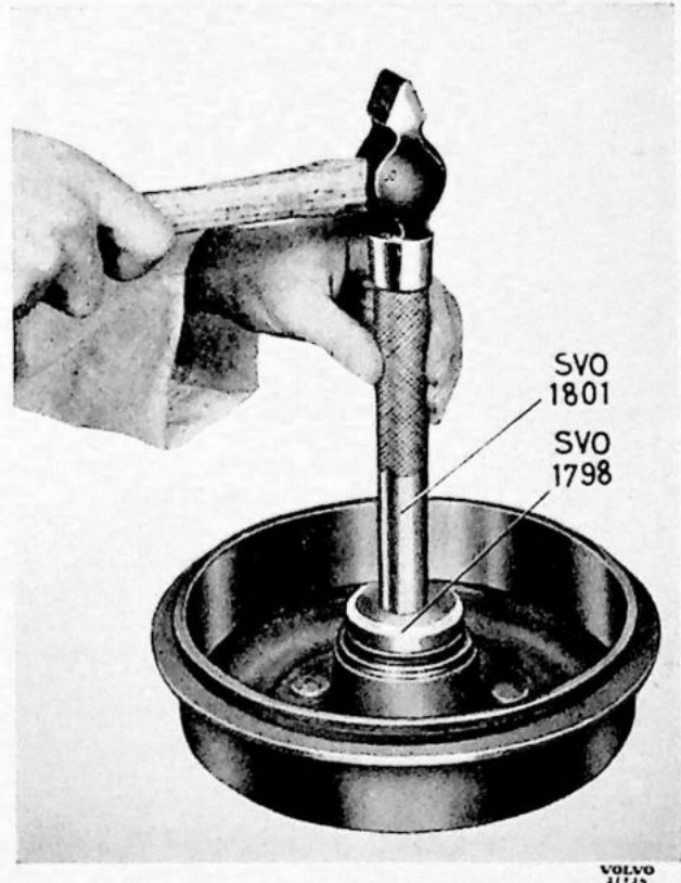
Fig. 9. Fitting the seal ring.
